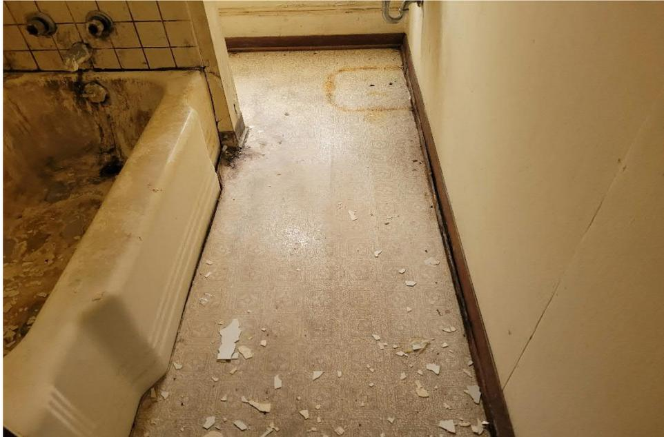
**Photo 5:** View of positive vinyl sheet flooring in bathroom of building 213 2<sup>nd</sup> floor apartment.
