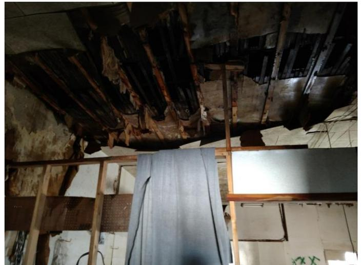
**Photo #10** View of first floor water damaged ceilings (building 213).
