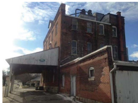
Looking south at the Property
