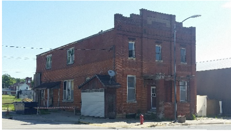
Side of Building
