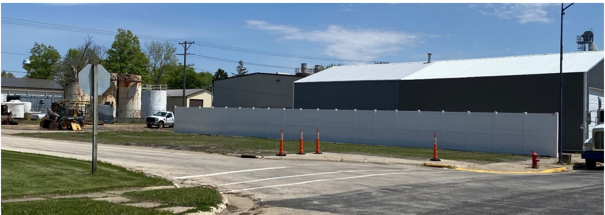
Site after Building demolished – July 2020
