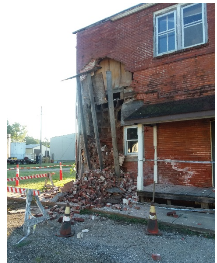
Back side of LeClere Building
