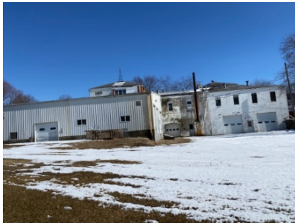
Back of Building (south side)
