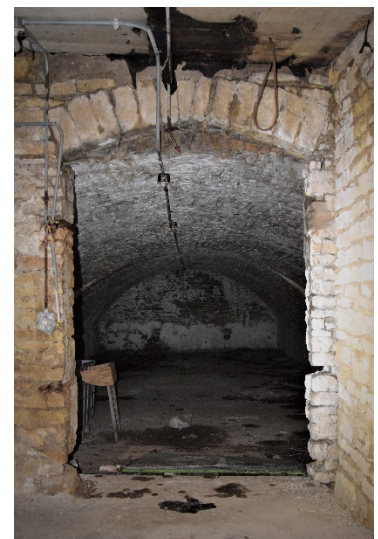
Beer Storage Vault
