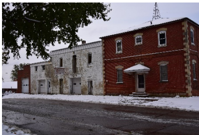
Close up view of front of building
