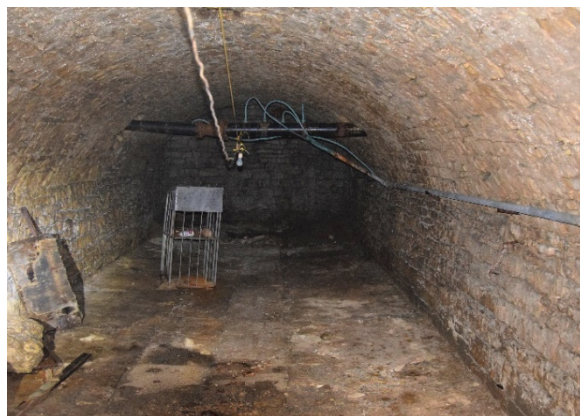
Beer Storage Vault
