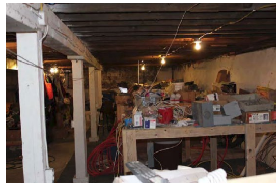
1004 S 4 th St. Basement
