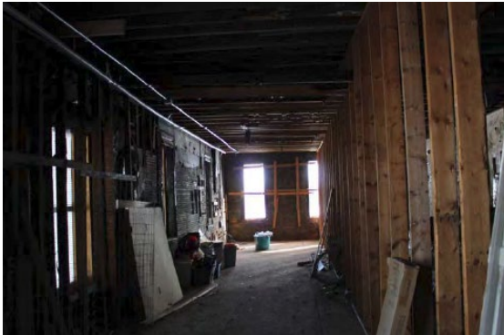
1000 S 4 th St Basement
